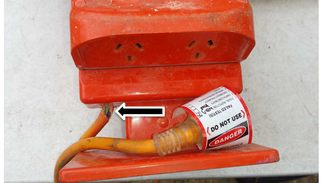
* Appliance MP021 FAILED - Damaged Lead
